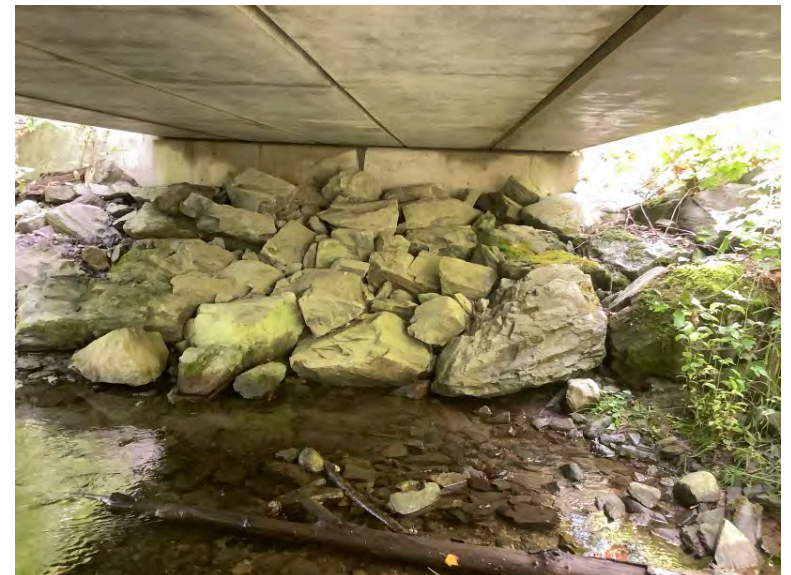
Right Bank Abutment when facing downstream
