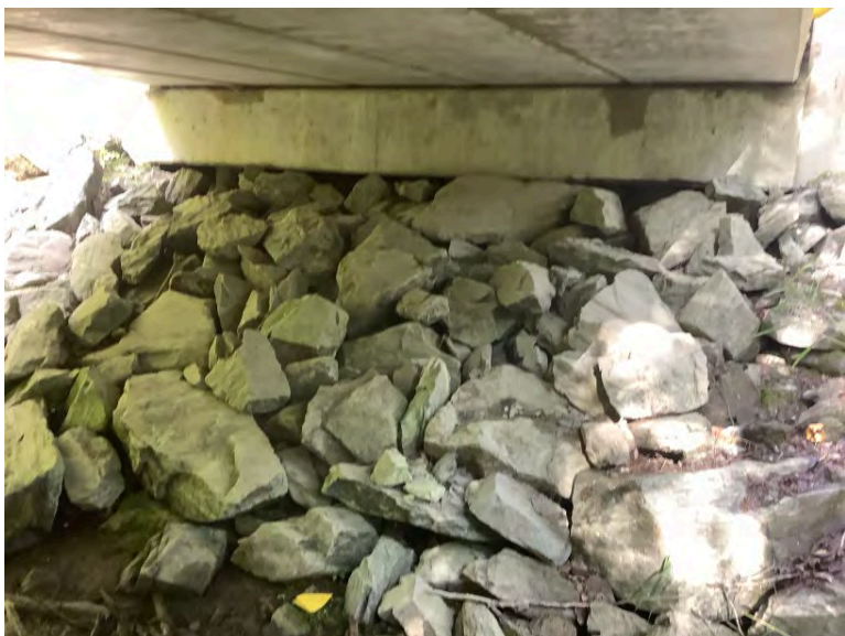
Right Bank Abutment when facing downstream
